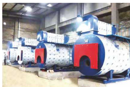
宁夏煤矿 6台10吨燃气冷凝锅炉 6 sets 10 t/h gas condensing boilers for Ningxia coal mine industry
