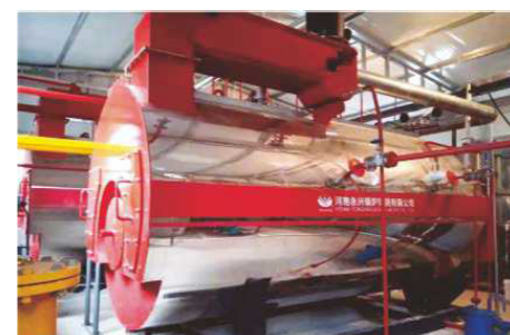
陕西延安洗涤行业 4吨低氮燃气蒸汽锅炉 4tph low nitrogen gas steam boiler for Shanxi washing industry
