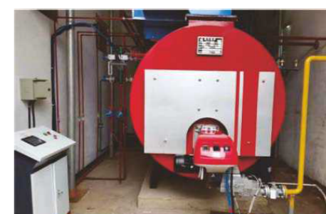
沈阳食品公司 2吨燃气冷凝锅炉 2 t/h gas condensing boiler for Shenyang food company
