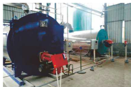
福建龙岩化工公司 4吨燃油蒸汽锅炉和180万大卡燃油导热油炉 4t/h oil fired steam boiler & 1,800,000 kcal oil fired thermal oil heater for Fujian chemical company
