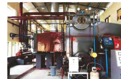
缅甸军工企业 15吨燃气蒸汽锅炉 15T gas steam boiler for Military enterprise
